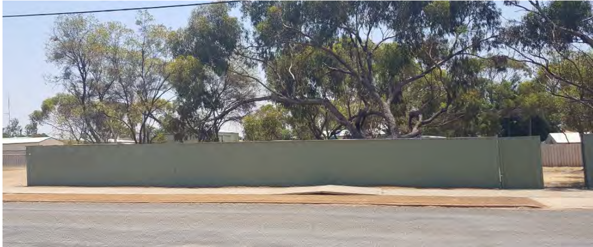
Figure 4.10: Examples of lifted, cracked or gravel covered paths
