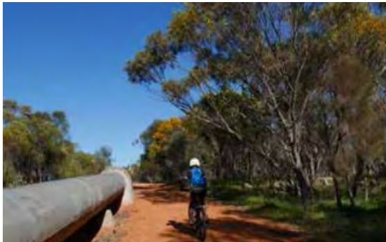
Figure 8.3: Trail along a Utility Corridor
