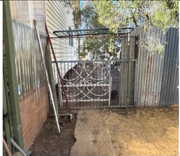
Access Gate Closed
