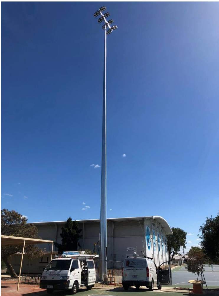
35m poles with 8no Sylvania Briteline Raptor LED fittings
