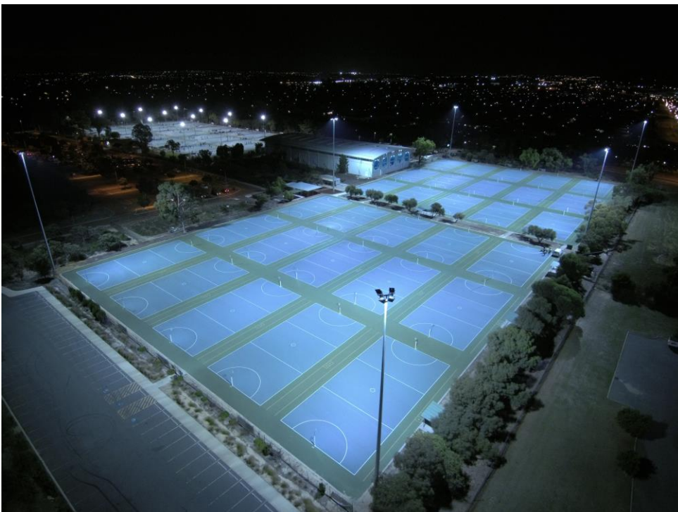
Drone photo of the commission LED fittings demonstrating exceptional uniformity asymmetric light cutoff
