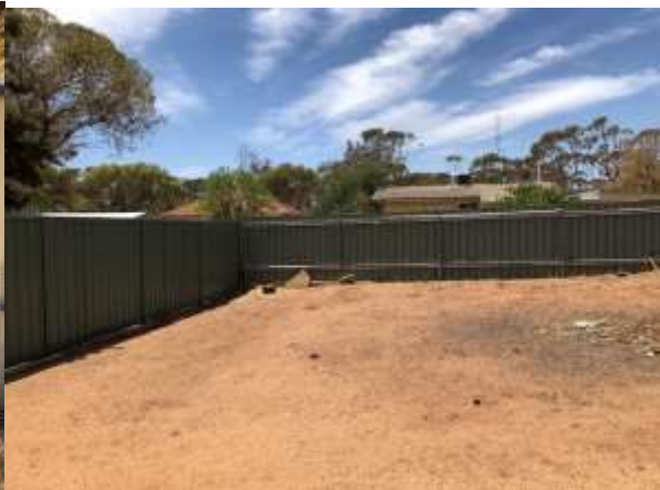
Fencing in back yard
