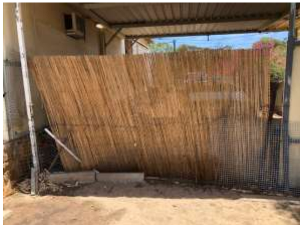
Dividing gate – under carport
