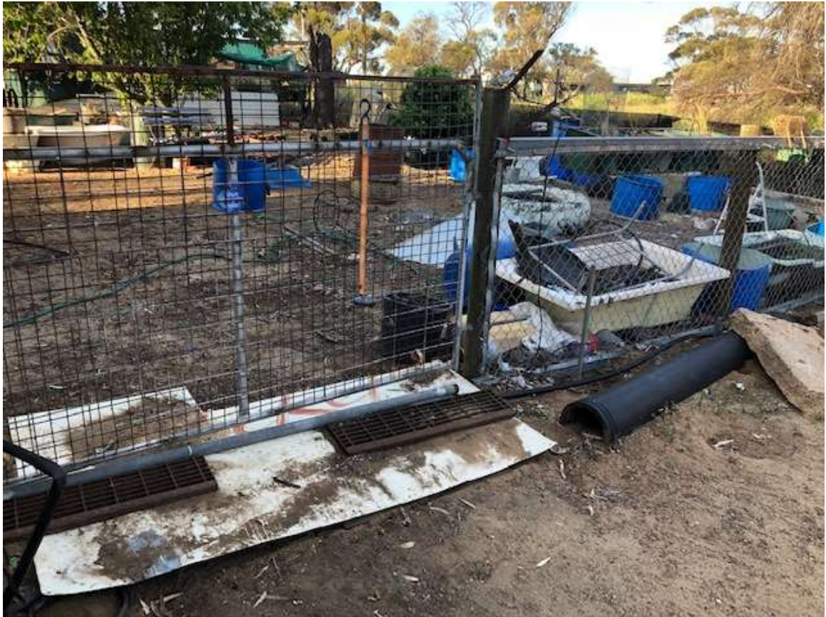
Fencing around yard
