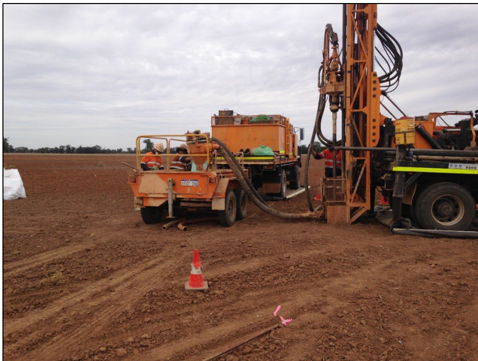
Figure 1: Zero Impact Trailer in Use at an Aircore Drill Site
