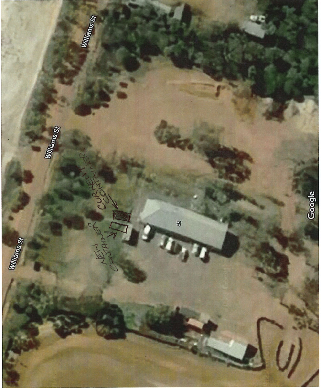
Goomalling Mens Shed 28 Williams Street, Goomalling
