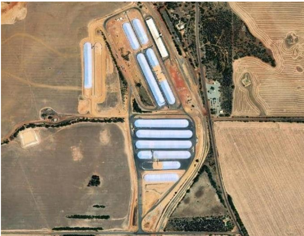
Figure 1 Overview of CBH Konnongorring facility
