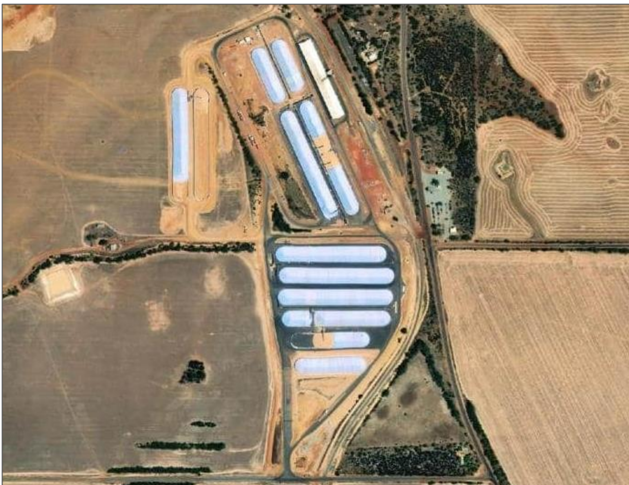
Figure 1 Overview of CBH Konnongorring facility
